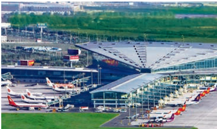
Tianjin Binhai International Airport
