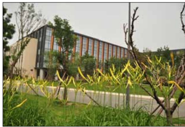
Huawei Digital Technology Co Ltd
