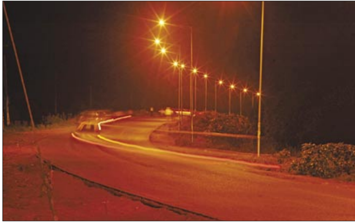
Streetlight projects throughout the city are making Nairobi Metro a safer place.
