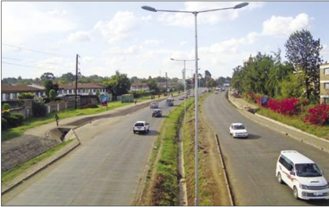
The 3-km Mbagathi Way street lighting installed by the Ministry of Metropolitan Development.
