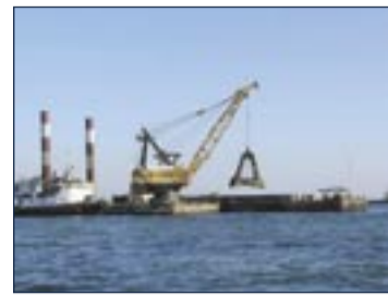
PROVIDED TO CHINA DAILY Construction at Dongjiakou Harbor
