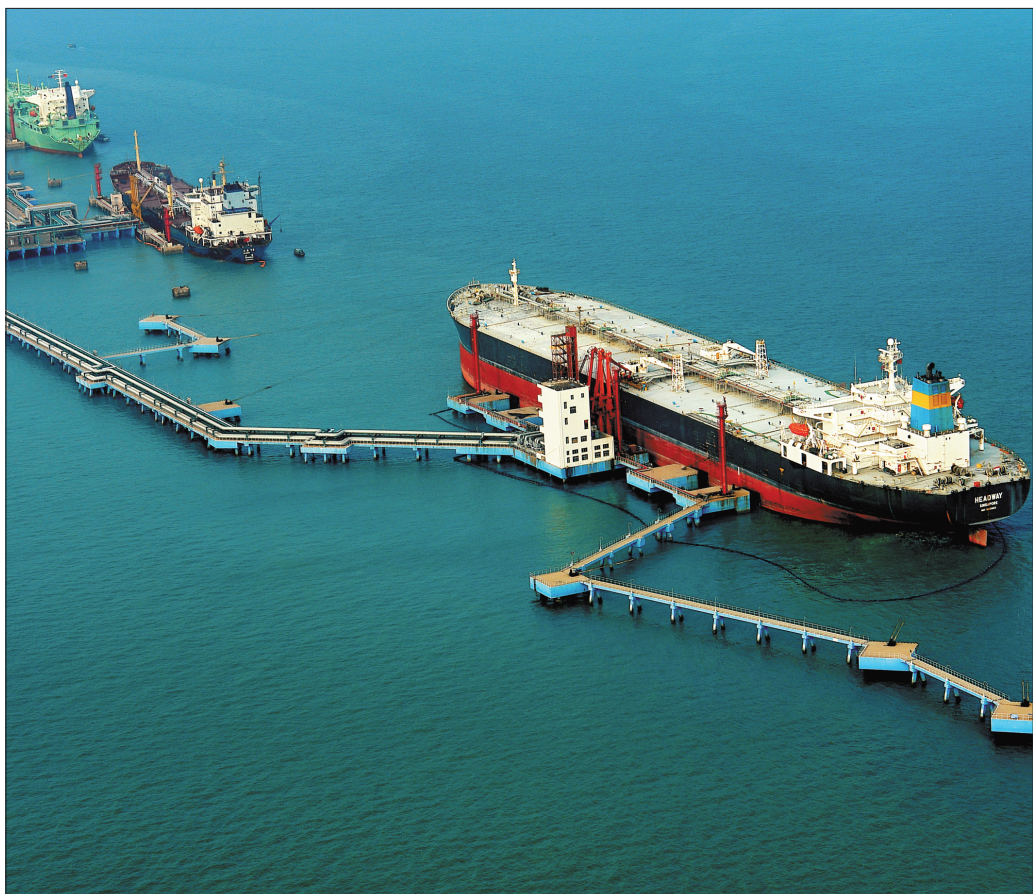
A petroleum terminal at Zhanjiang Port. The port handled more than 200 million tons of cargo last year, making it one of the leading ports in Guangdong province.
