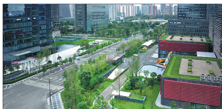
A glance of the Chengdu Financial City. The area, covering five square kilometers, is under construction. It is expected to become West China's financial hub.
