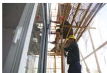
Workers are busy installing elevators in a residential building. — Fu Tianhao
