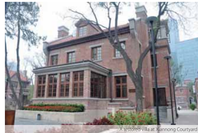
A restored villa at Xiannong Courtyard
