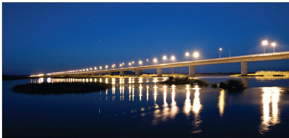
Bridge over the Zambezi River at the city of Tete.
